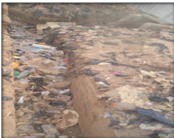
Non-biodegradable waste in drainages in the study area
